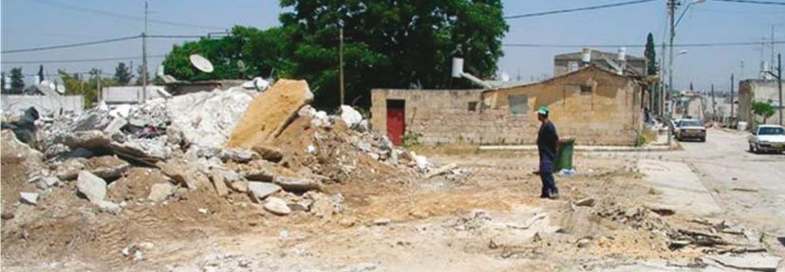
Demolition of houses in Remez neighborhood, Lod, 2005
