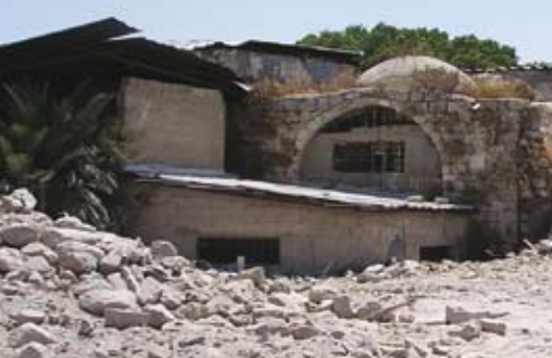
Demolishing Ramle's Armenian neighborhood, 2003
